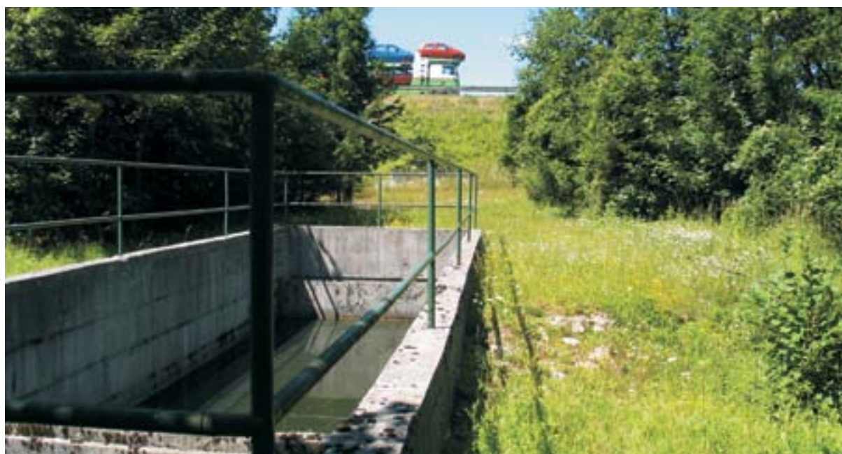
Fig. 1: Rainwater that washes the roadway of the motorway runs off into the oil collector, where in favourable conditions of small inflows sedimentation occurs. On the other side of the oil trap the water drains directly into the karst. Fluorescent tracer was injected into the drainage shaft of the oil trap (Gabrovšek et al. 2010).
