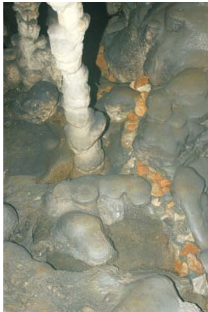
Fig. 2: Electric cable protected and masked by concrete at Kalvarija.
